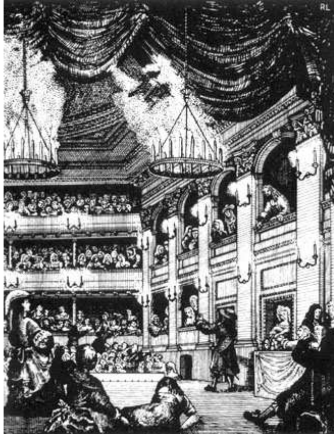
Restoration drama in progress
